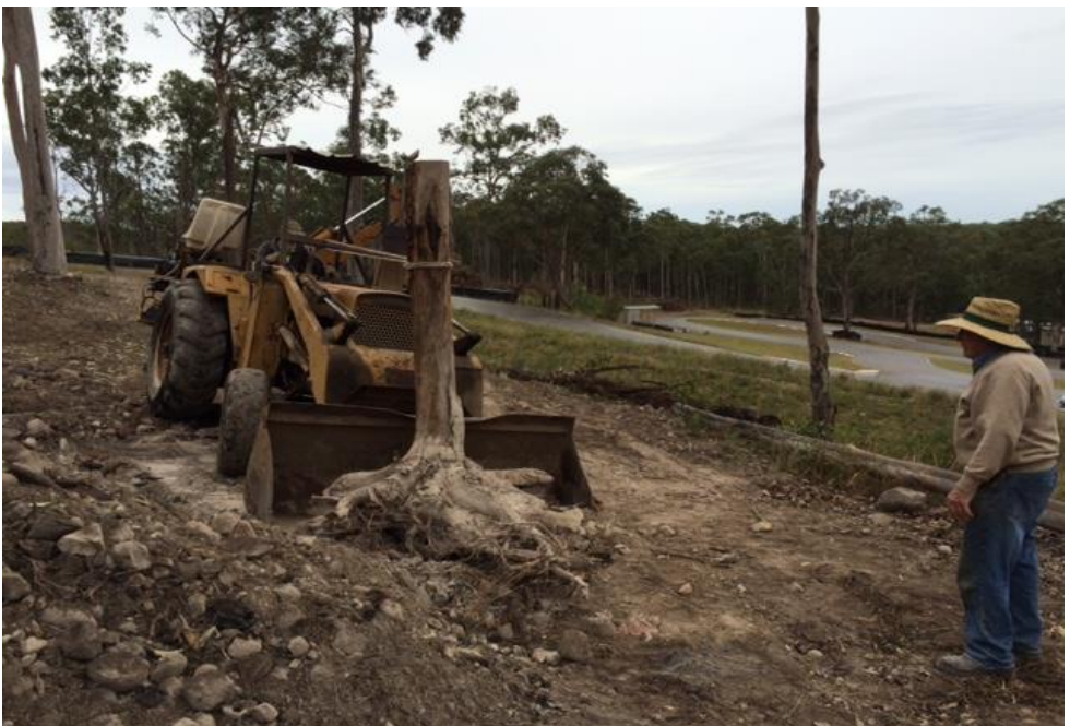
Below: On going work out at Ringwood Park.
