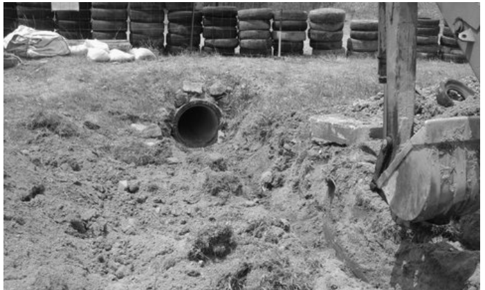
The start of the drainage extension to accommodate the new finish.
