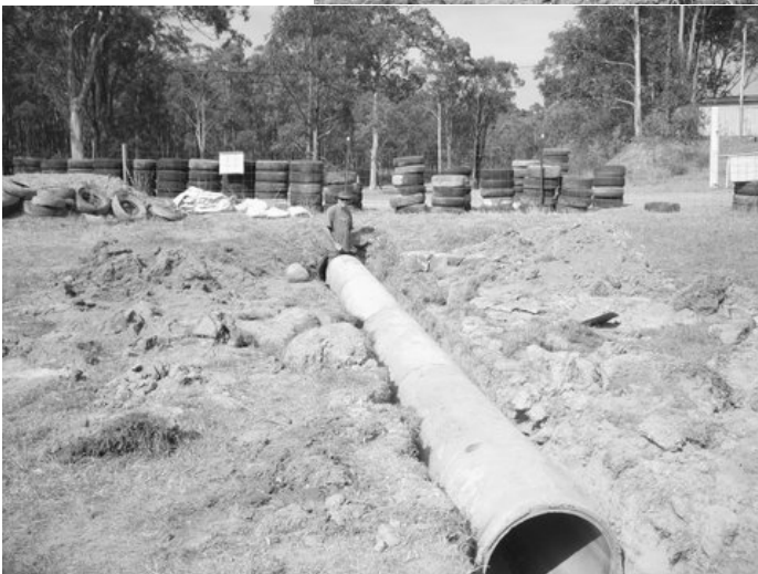
Pipes laid, ready for fill and headwall construction.
