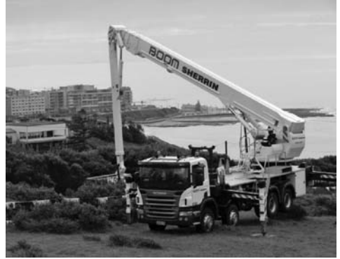
Cherry picker in place
